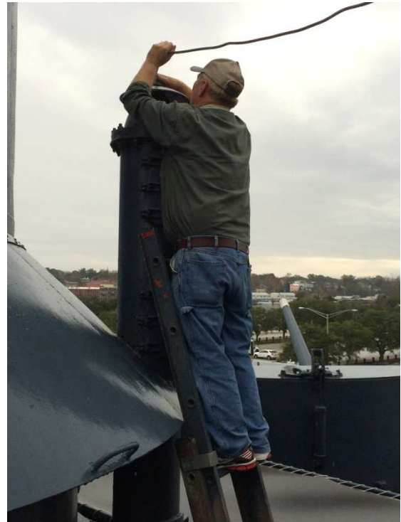
Linwood Todd (NT4F) troubleshooting one of the antenna lines on board the USS North Carolina (BB-55)
